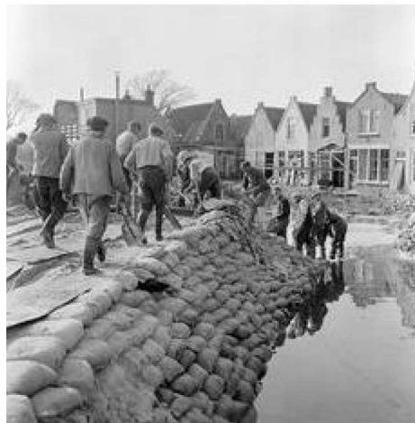
Photograph 9.3. Cooperation to build dikes after the great storm of 1953
